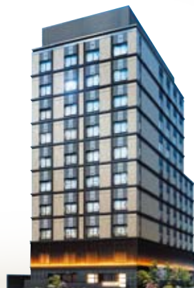
Mitsui Garden Hotel Kyoto Station
